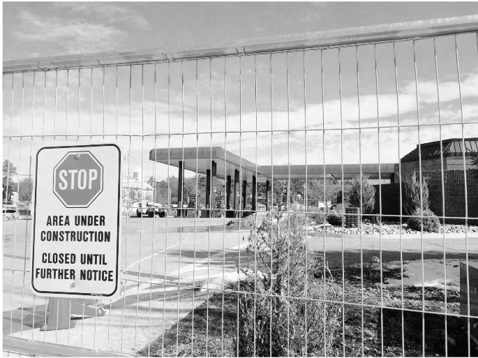
A metal fence surrounds the closed Sheetz at Shiloh Road and Benner Pike on Monday.
