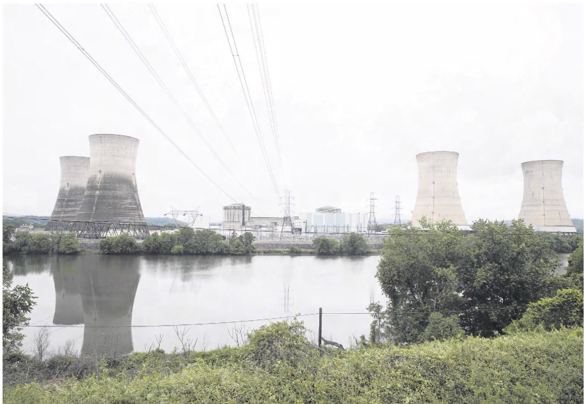
On June 1, Exelon Corp. plans to begin the monthslong process of shutting down the financially struggling Three Mile Island nuclear power plant in Middletown, which was the site of a partial meltdown in 1979.
