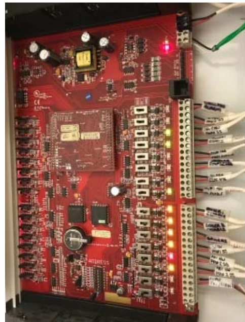
Control circuit board for three boilers and two chiller units.
