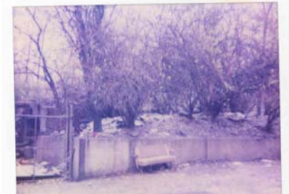
Crack Forest before cleanup
