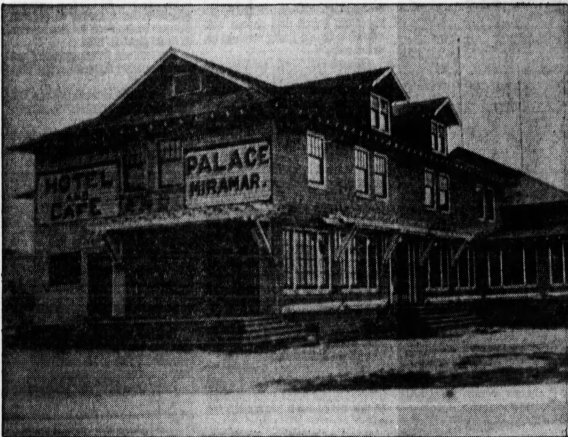
The Miramar Hotel as it appeared in the 1920s, when run-runners made Coastside a legend
