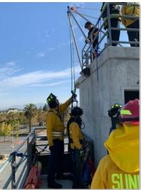
such as a large tree or I-beam at the scene of a rescue. Because it is portable, the Vortex can be deployed in a variety of rescue scenarios. In the urban environment, the Vortex can be well suited to mitigate difficult situations such as a blind-shaft elevator rescue by serving as both a high directional system, and anchor point. For more information please contact Captain Ryan Yin at ryin@sunnyvale.ca.gov.
